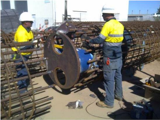
*Fixing O-cell Assembly to Cage*
