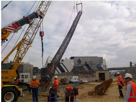
*O-cell Instrumented Pile Cage Being Lifted*
