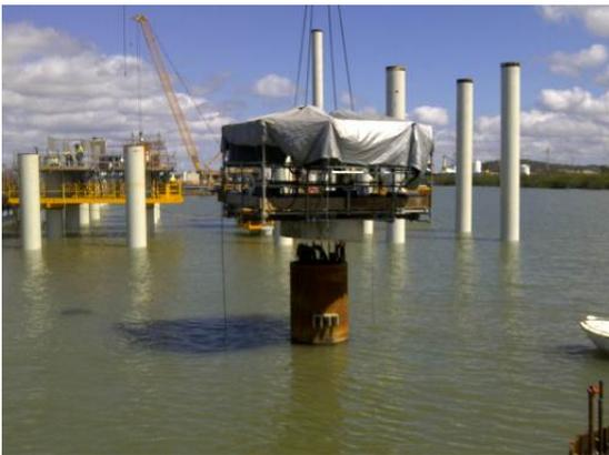
*Testing Platform Being Lowered on to Pile*
